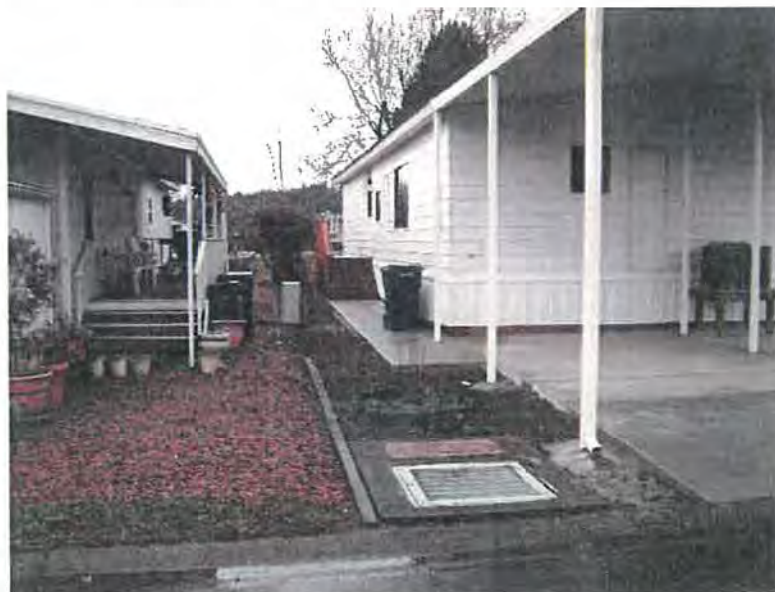
SIDE VIEW - LOOKING AT WEST SIDE OF BUILDING - Photo Taken 03-04-2014
